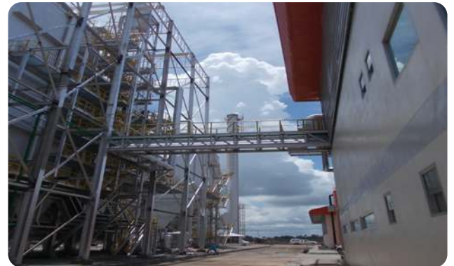
17 MW Rice Husk Fired Power Plant, Surin Province
