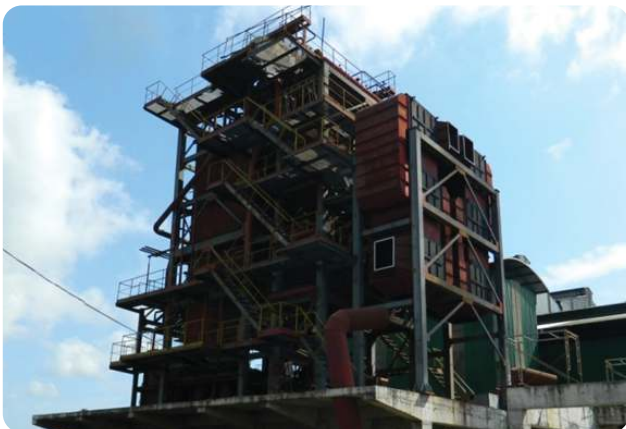
2.4 MW Empty Fruit Bunch/Palm Fiber Fired Power Plant, Surat Thani Province
