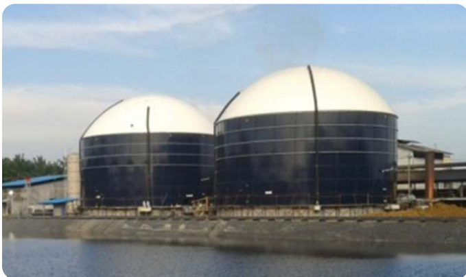
Two Stages Reactor for Biogas Production from Palm Oil Mill Effluent (POME)
