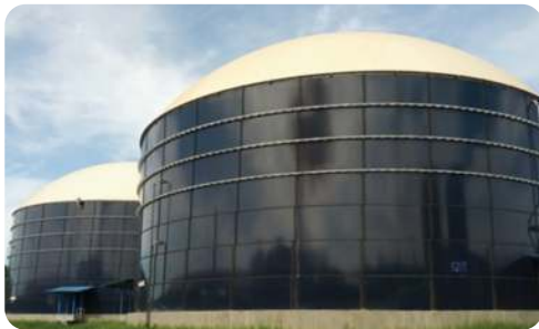
Bolted Glass-Fused-Steel CSTR
